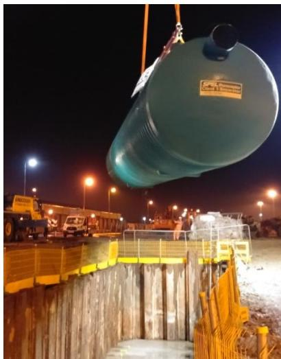
Up to 4.4 hectares of hardstanding area, with a rainfall of 65mm per hour, can be treated to meet less than 5mg/litre of hydrocarbons in the outlet under the standard test conditions of the European Standard.
